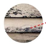
Blistering and/or peeling of outside paint Possible cause: Excessive moisture or high humidity due to poor attic ventilation
